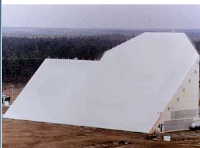
The AN/FPS-85 phased array radar at Eglin AFB, Florida, is an element of the Space Surveillance Network (SSN) that detects, acquires, correlates, and tracks space objects. Source: Federation of American Scientists.
