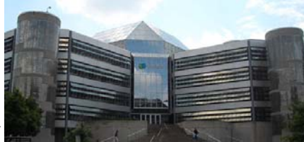
Intelsat headquarters in Washington, DC.
